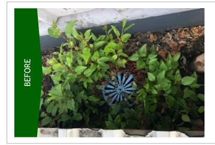
The gutters to the roof were in quite a bad condition, with high levels of debris, silt and vegetation in the gutter valleys, most of the outlets where obstructed or completely covered. Little or no maintenance can cause the gutters to become overwhelmed by vegetation which is return causes excessive weight on the gutter boxes which can open the box gutter joints causing leakage and water ingress, the moisture and standing water can accelerate corrosion.
