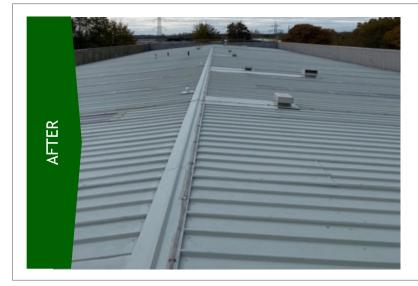
The preparations to the roof started with a jet clean to remove all debris and loose coatings, once the roof was clean and clear we began to treat the corrosion. The corrosion treatments included mechanically abrading the substrate to remove the surface corrosion and any gingering.
