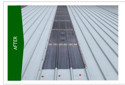
The redundant lights not required where over-sheeted using steel roof sheets to match the profile, these were fixed down and sealed using butyl sealants to leave watertight.
