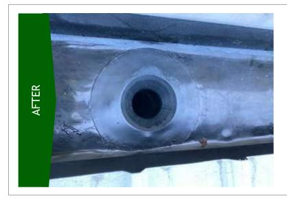
In order to fit the new liners in to the box gutter channels all debris had to be cleared, bagged up and removed from roof level down into the site skip, once the gutters had been cleared any remaining outlet guards where removed and placed to one side.
