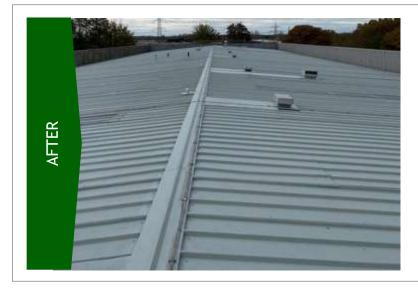
The preparations to the roof started with a jet clean to remove all debris and loose coatings, once the roof was clean and clear we began to treat the corrosion. The corrosion treatments included mechanically abrading the substrate to remove the surface corrosion and any gingering.
