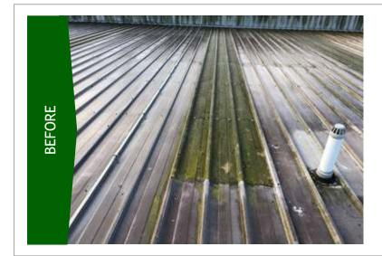
The existing GRP roof lights where covered by organic matter and had started to completely breakdown due to UV exposure and general weathering, the condition of the sheets stopped any type of day light transmitting into the areas below.
