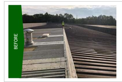
The composite roof was heavily soiled due to little or no maintenance over the years, the original factory applied applied coated had started to fail with loose and flaking coatings throughout, with corrosion to the panel profiles and cut edges of the ridge, hip flashing and soaker sheets.
