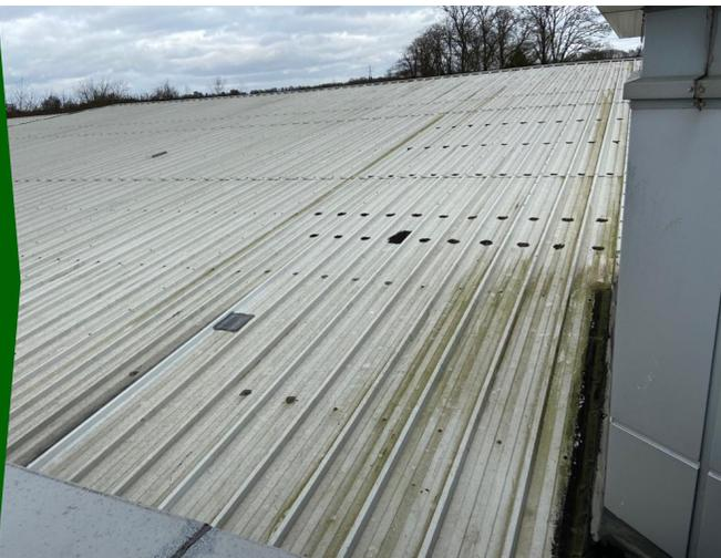
The existing roof sheets were dirty and there was evidence of historical patch repairs throughout, cut edge corrosion was present on the sheets which had caused the original factory applied coatings to start peeling back exposing the steel substrate.
